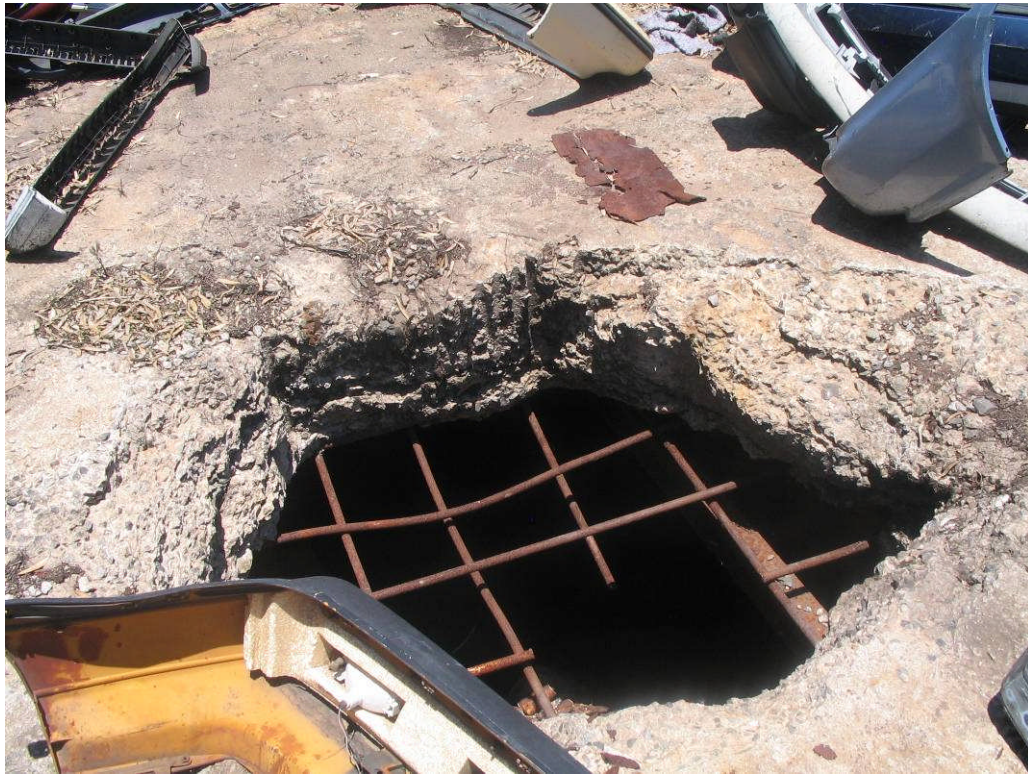
Figure 4.12. Access attempt through reinforced concrete seal, Kleinfontein Mine (Ekurhuleni)
