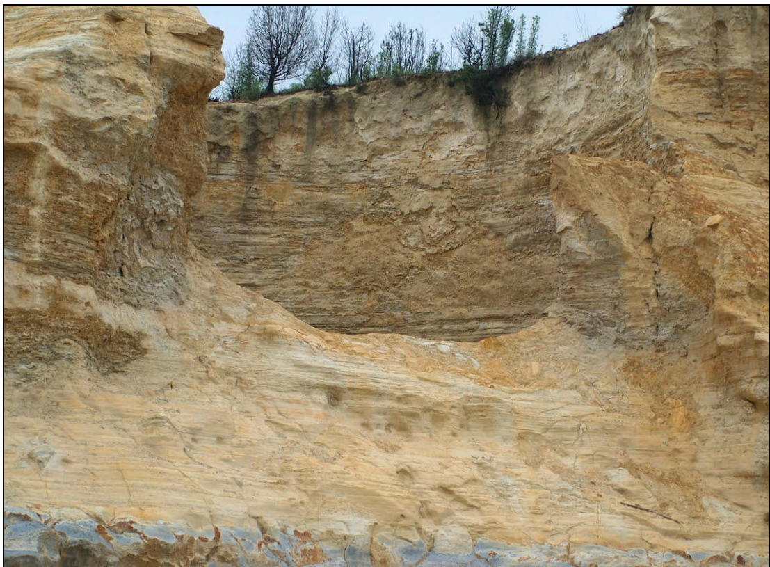
Figure 3.6. ERPM24x, collapse of a slimes dam into an underlying mine opening, Ekurhuleni
