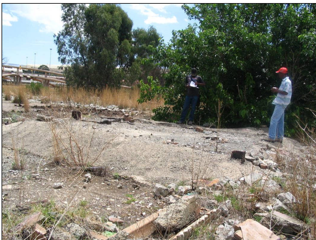
Figure 4.11: Typical shaft sealed with concrete seal (Crown Mine 8 Shaft A, Johannesburg)
