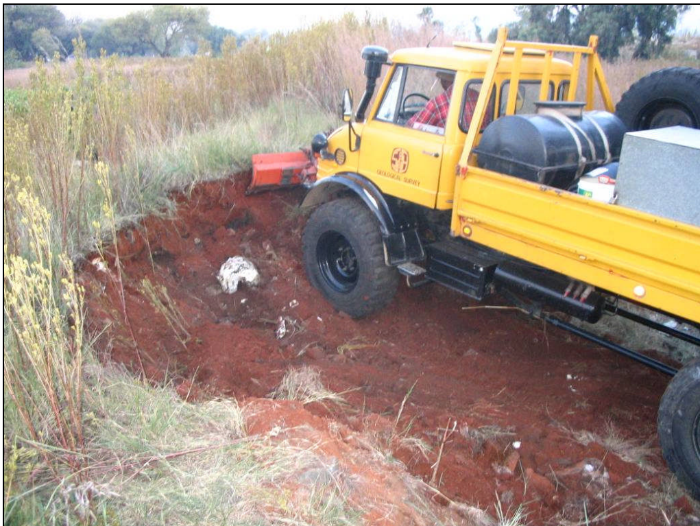
Figure 5.7: Placing covering material over PUF filled shaft
