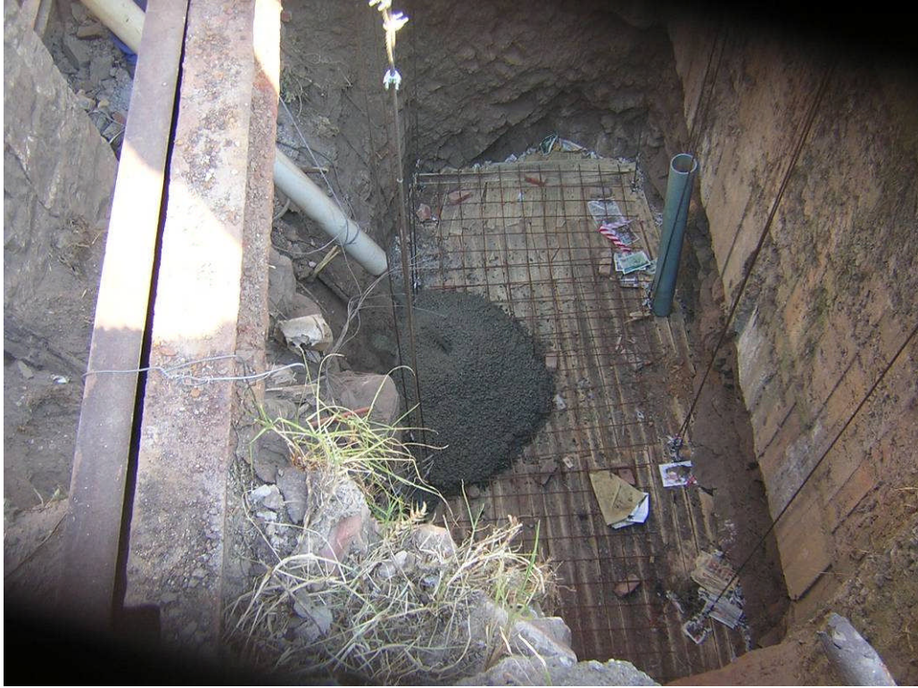
Figure 5.14. Sacrificial formwork, suspended by steel cables from steel girders, prior to the casting of the primary slab
