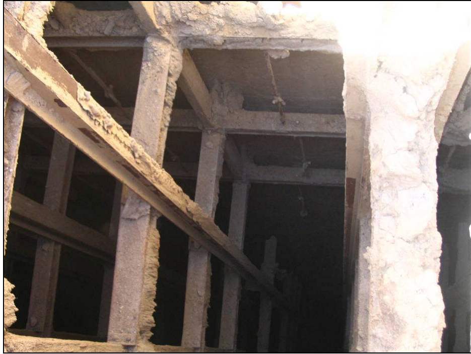
Figure 1.6 Steel framework within an abandoned, vertical mine shaft (Rand Leases Mine, Roodepoort)
