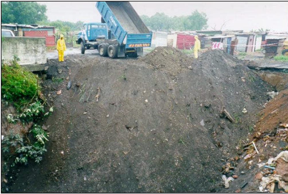
Figure 1.11: Uncontrolled backfilling, Boksburg (circa 2004)
