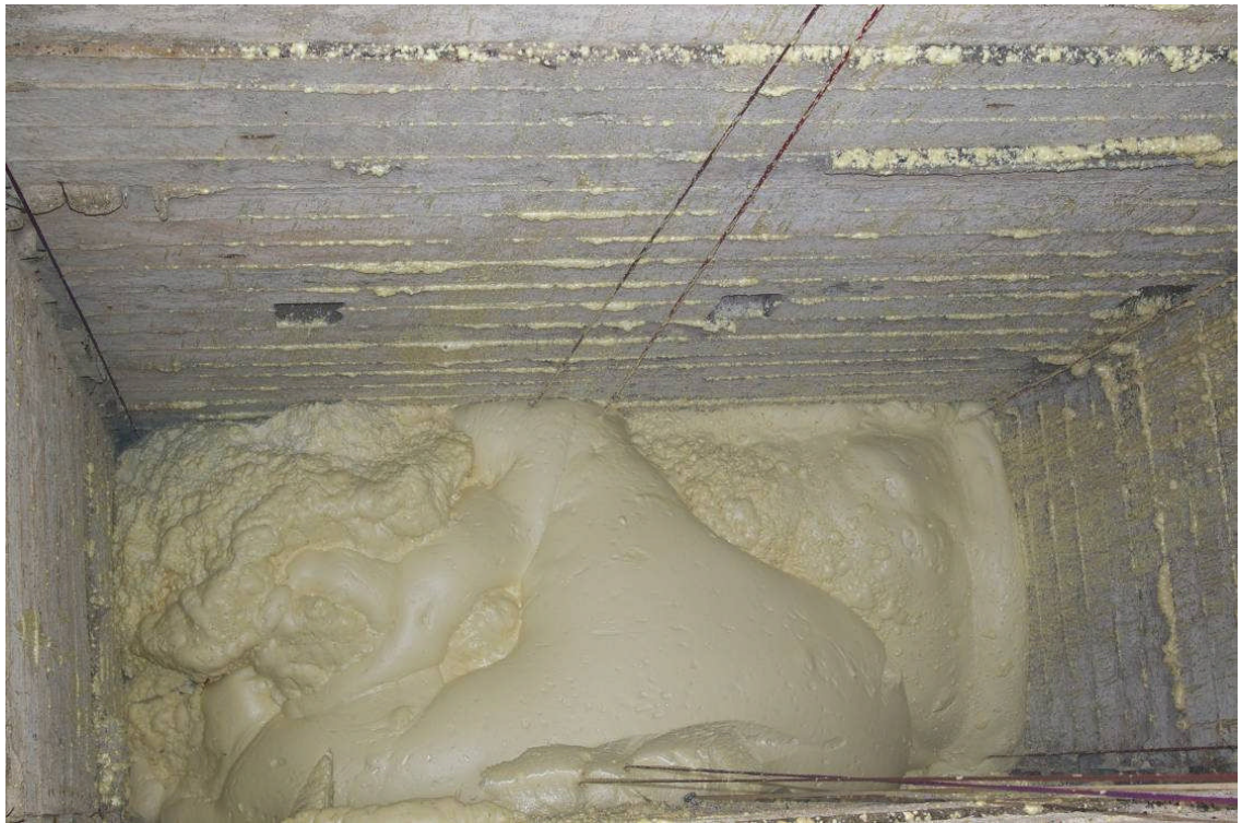
Figure 5.9. S & J 15B: PUF plug being created in mine shaft
