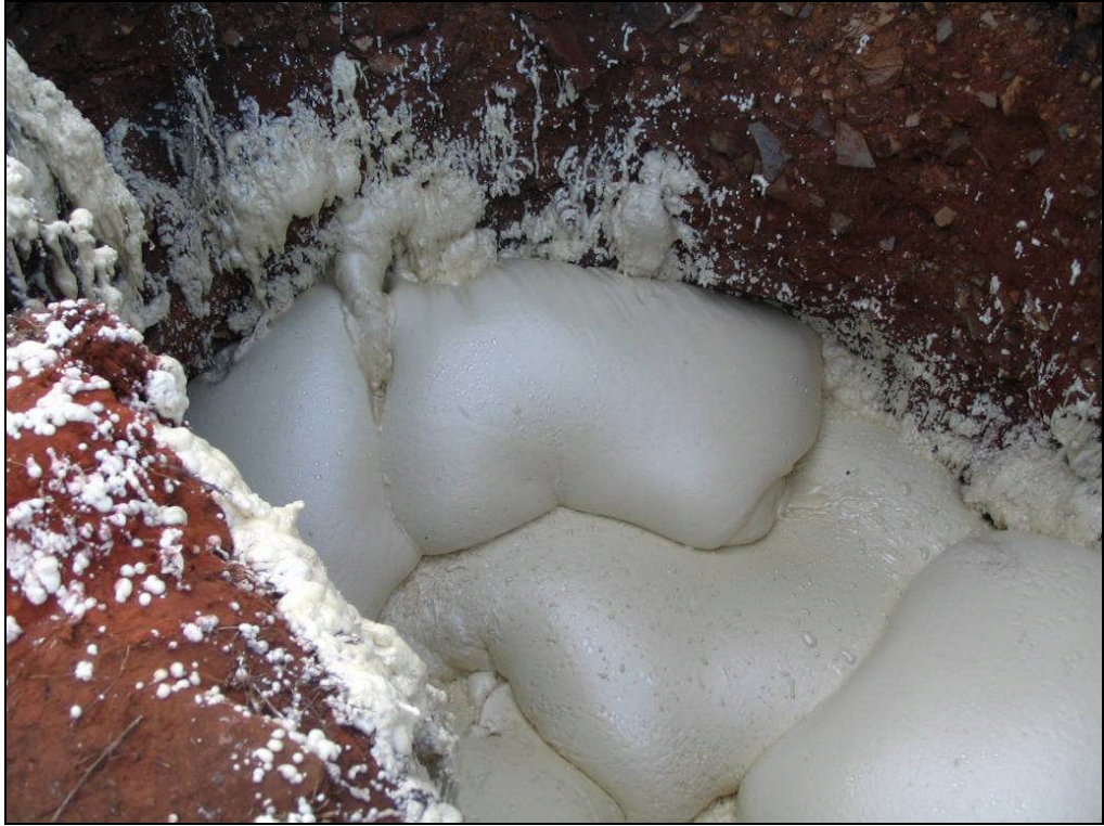
Figure 5.6: Layers of expanding foam
