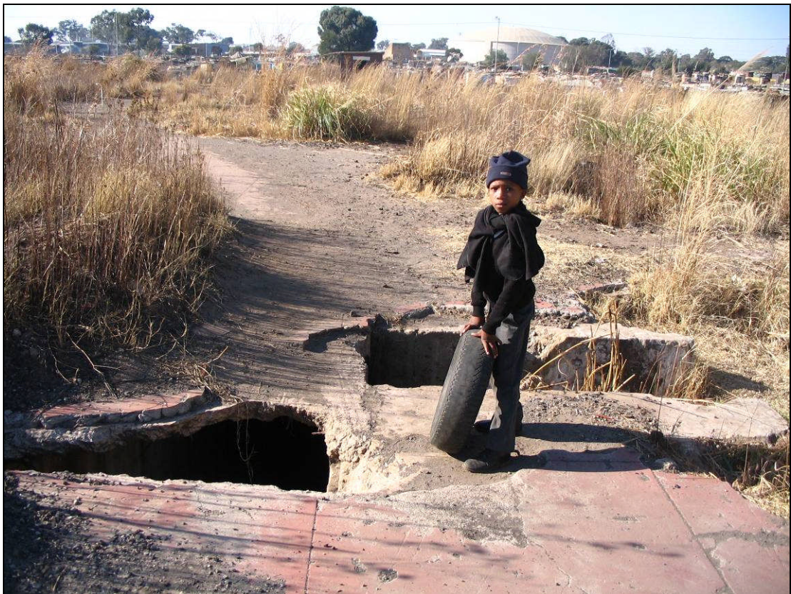
Figure 1.1 Local inhabitant dangerously close to two abandoned mine shafts, Johannesburg. Each of these openings is believed to be approximately 500m deep.
