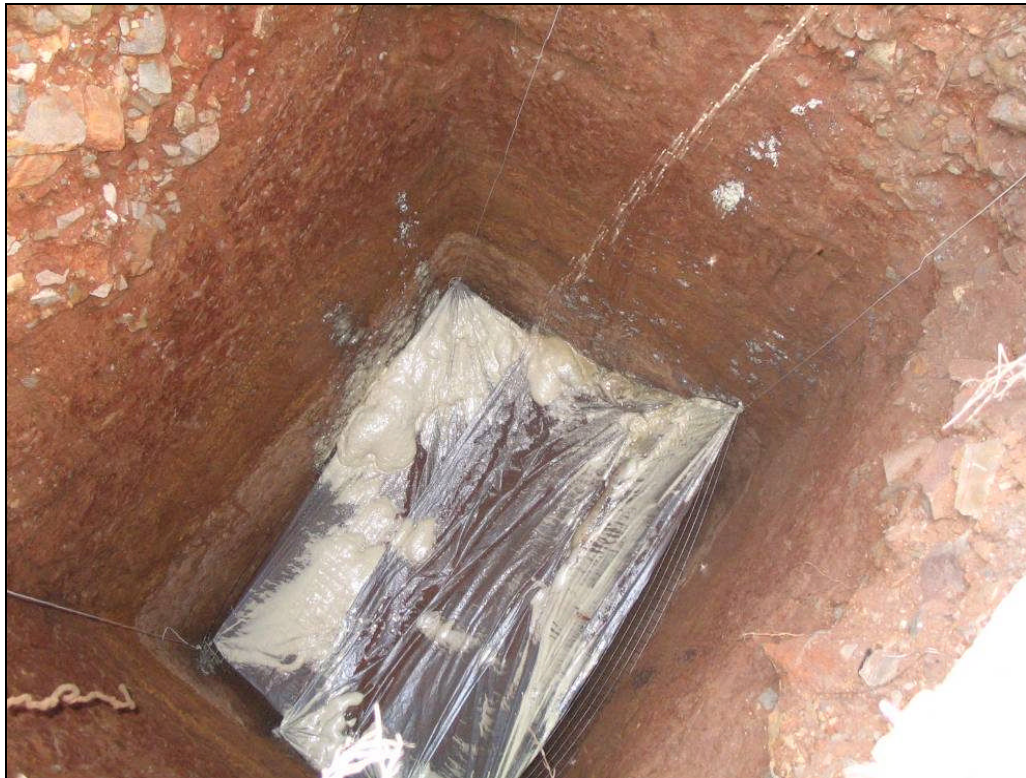
Figure 5.4: Base of plug being lowered into position
