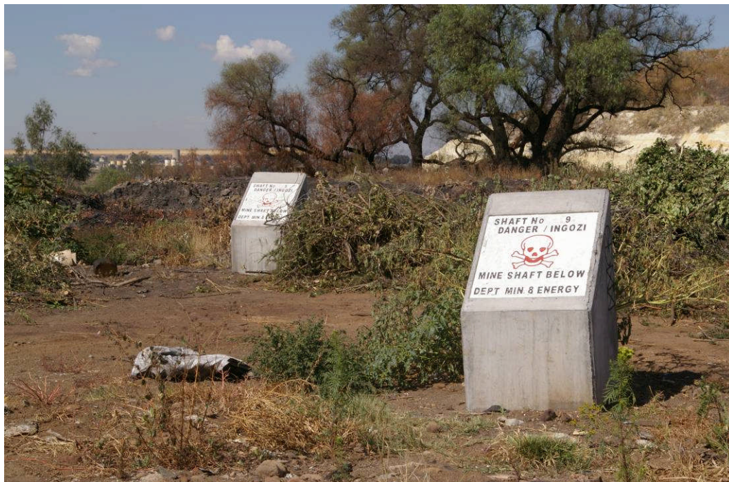
Figure 5.17. Typical landmark placed on sealing of a mine opening
